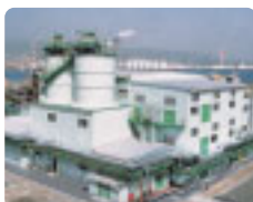
Plant to turn incinerator ash into raw material for cement
