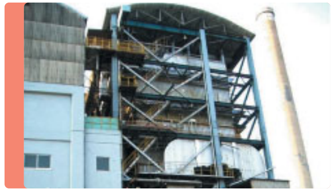
No. 2 power plant with waste wood mixed fuel-burning demonstration facility
