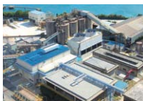
Waste heat recovery power generation system at Kanda Cement Factory (Cement and Construction Materials)
