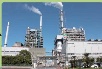
IPP, in-house power generation
