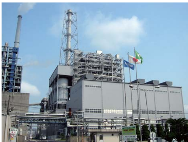
IPP power plant
