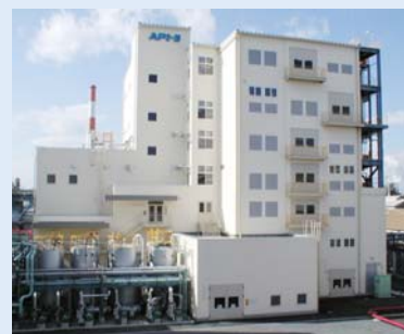
AP-3 manufacturing facility
