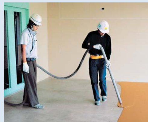
Application of self-leveling materials
