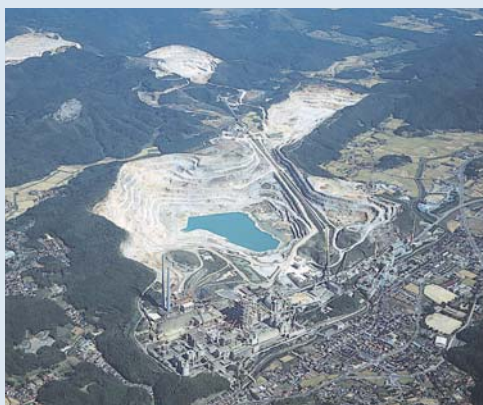
Isa Cement Factory and limestone mine
