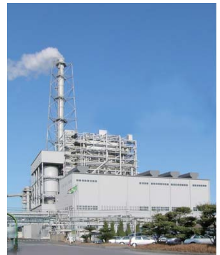
IPP power plant
